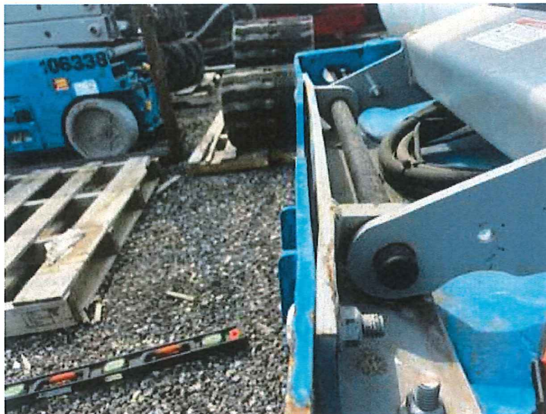
Figure 2: Bent Lower Lift Stage Mounting Bracket.
