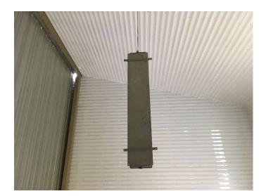
One of the lights in the clarifier building has become dislodged from its ceiling attachment and is hanging by its wire. This should either be reattached or disconnected prior to moving the wastewater treatment plant to its final location.
