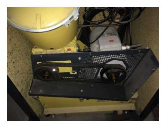
The acoustic enclosure on the process air blowers on bioreactor skid 1 and skid 3 were both removed at some time prior to inspection. And one of the blower enclosures has suffered some minor cosmetic damage.
