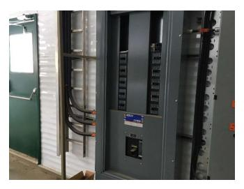
Apart from seemingly missing the breaker cover panel and accumulated dust. The main power panel appeared to be in excellent condition.
