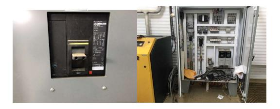
Its recommended that the electrical panels be blown out with dry air prior to being placed into service.
