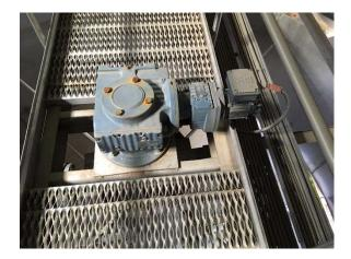
Like the feed pumps, all of the sludge return pumps had noticeable scrapping' noise and feel when the rotated by hand likely indicative of some bearing damage. These pumps should definitely be inspected by a millwright to ensure alignment and to inspect/replace bearings and seals.
