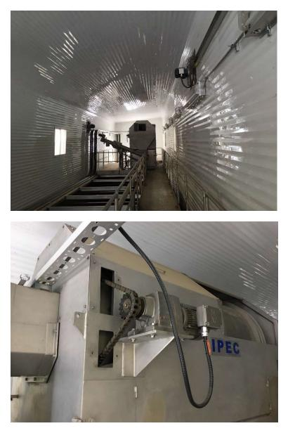
The screenings washer/compactor receives the raw screenings from the rotary drum screen. The screenings washer/compactor has a connection to the system potable wash water system and washes the raw screenings to remove organics prior to compaction and discharge to a storage bin.
